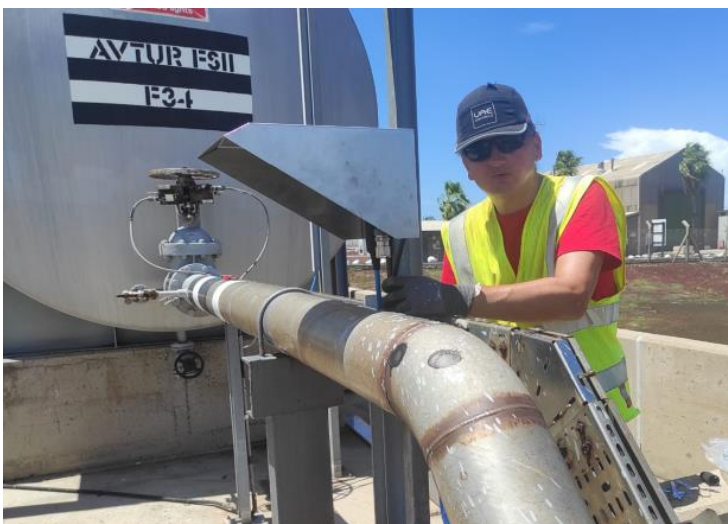
Connection of cabling for new ATG at Ascension
