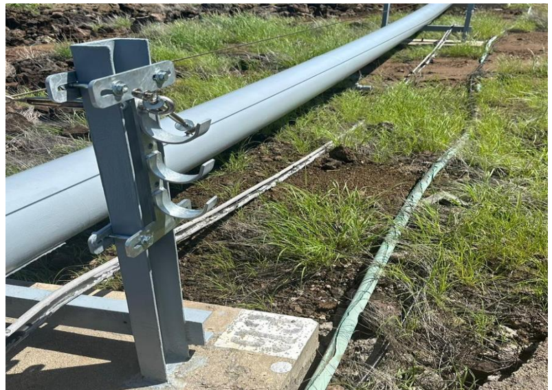
Repaired 10" pipeline support with cables holder at Ascension
