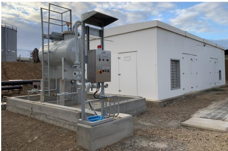
Ascension fire pump station after repair
