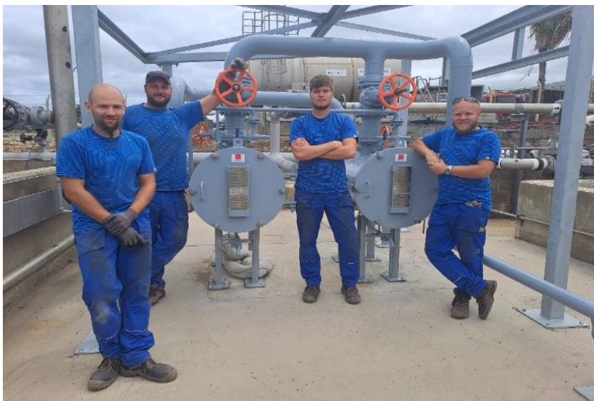
VAE staff at Ascension after commissioning of microfilters
