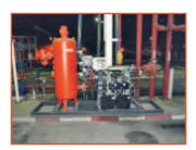
Unloading skid with vertical deaerator complete with multi-point level monitoring, providing total elimination of air from the product.
