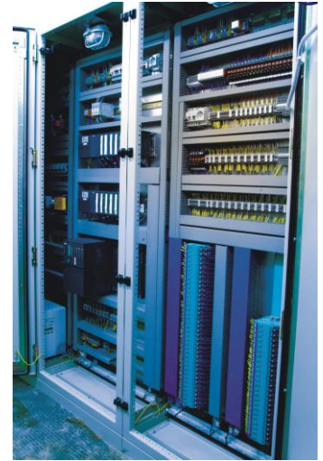
Electrical panel with PLC system
