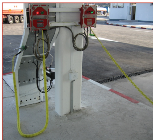
Two of EGT 4 with coiled sensing cables
