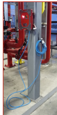
EGT 4 with straight sensing cable
