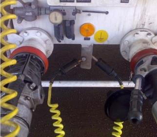
Shell terminal in Helsinki airport is used for loading of tank truck which distribute the aviation fuel to the aircrafts. For ensuring secure function it became necessary to test whether the tank trucks are correctly grounded.
