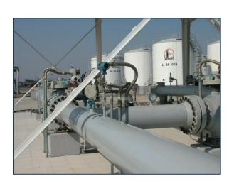
The reconstructed terminal is equipped with twenty new bottom loading arms suitable for diesel and petrol loading. Each arm is equipped with highly-precise additive dosing unit EVA6, a product of VAE CONTROLS. Stand-by gear pumps guarantee extremely high reliability and serviceability of the additive supply system. The new facility is controlled by new automation & dispatching system, which ensures local automation and integration of specific parts of the system
