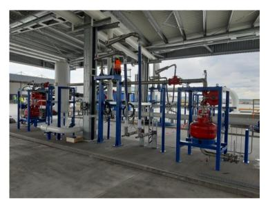
The implementation included delivery of a new control system, measuring lines (SKIDs) with flow computers Accuload IV, including metrological verification (MID). The delivery and installation of switchboards, cable routes, cabling, field instrumentation was part of the project. New TAMAS dispatcher licenses and SCADA visualization were implemented. This included start-up, commissioning, calibration and local staff training.
