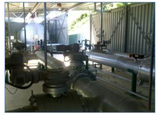
Roudnice ensures storage of diesel fuel for mimitary purposes in underground steel tanks witch capacity 5000 m³ each. The tanks are filled through product pipeline. Tank trucks loqading terminal is equipped with bottom loading arm located in special steel house underground for high secirity against attack. Tankfarm and tanktruck terminal are constructed in accordance with all NATO standards.
